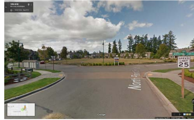
① VIEW OF SITE FROM EAST (139TH ST SE)
